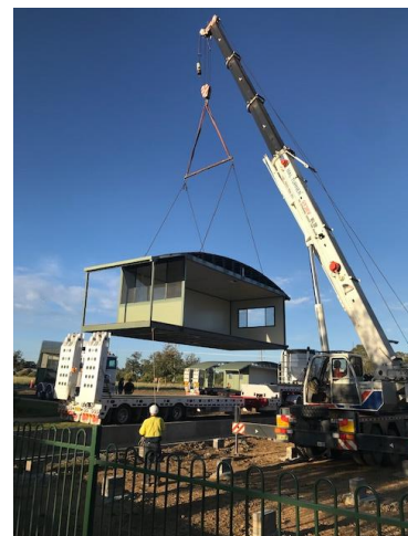
New Building Complex arrived in January
