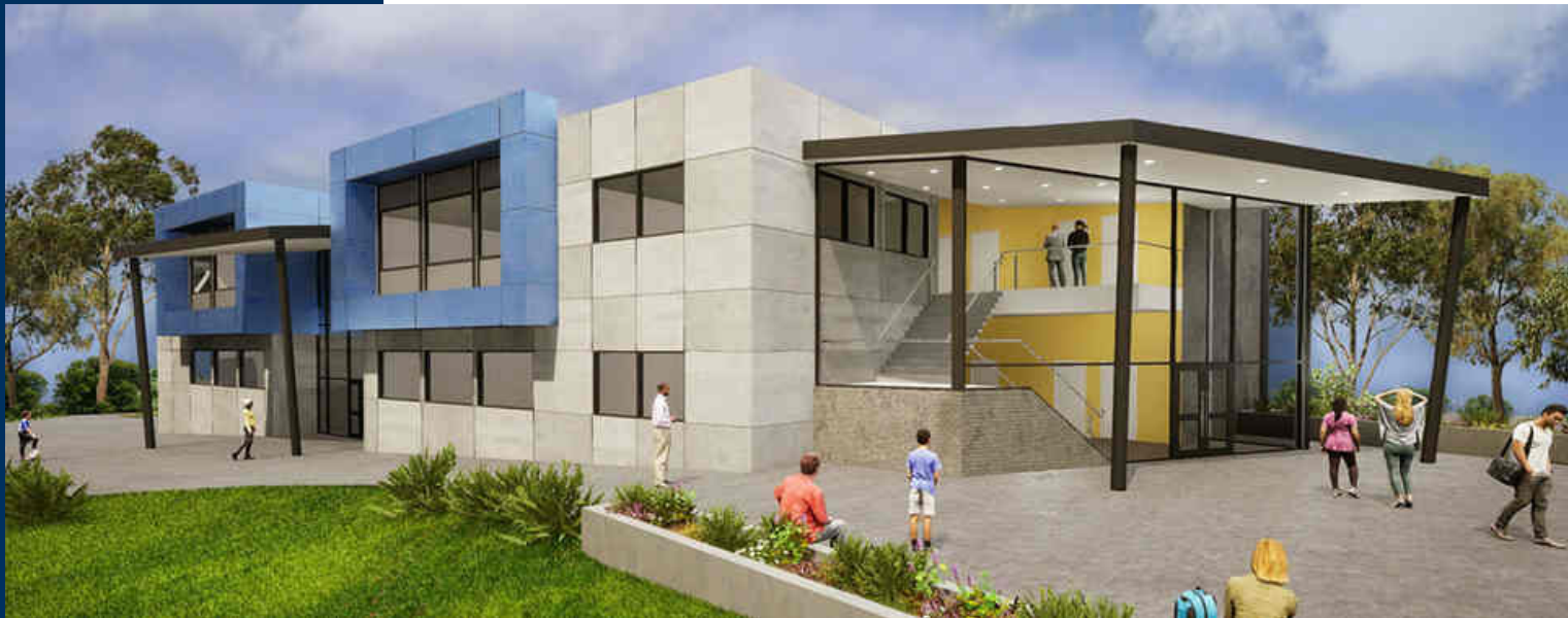
Senior School Building
